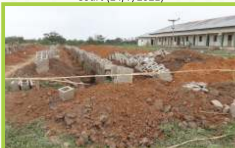
Block setting of the newly constructed female hostel at Igbaja campus (1/8/2021)
