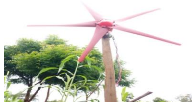
Figure 2: Showing a mounted turbine
